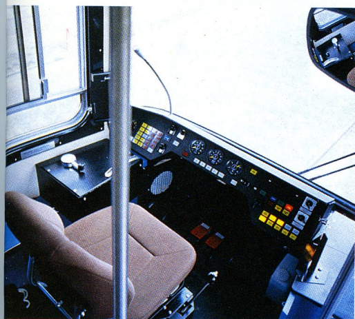
All necessary switches, signal lights, and meters as well as the controls for the loudspeaker and radio-telephone equipment are mounted in the driver's desk. The controller is to the left and the parking and emergency brake switch to the right of the driver.
